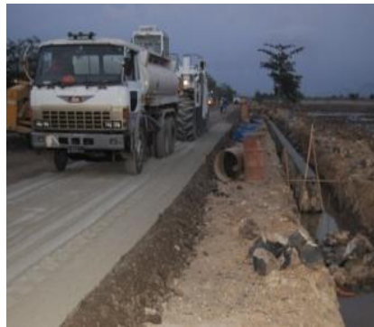
Proses recycling aspal
