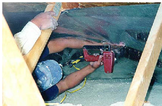
Figure 113—Installing Radiant Barrier
