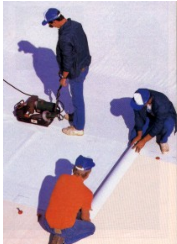
Figure 110—White Single Ply Membrane with Heat-Welded Seams
